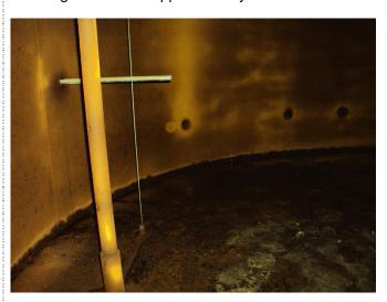
The floor and wall of the tank was uncoated carbon steel and had been inspected in the last 10 years. No pH checks were carried out as part of this inspection. The inspection concluded that the tank was in good condition.
